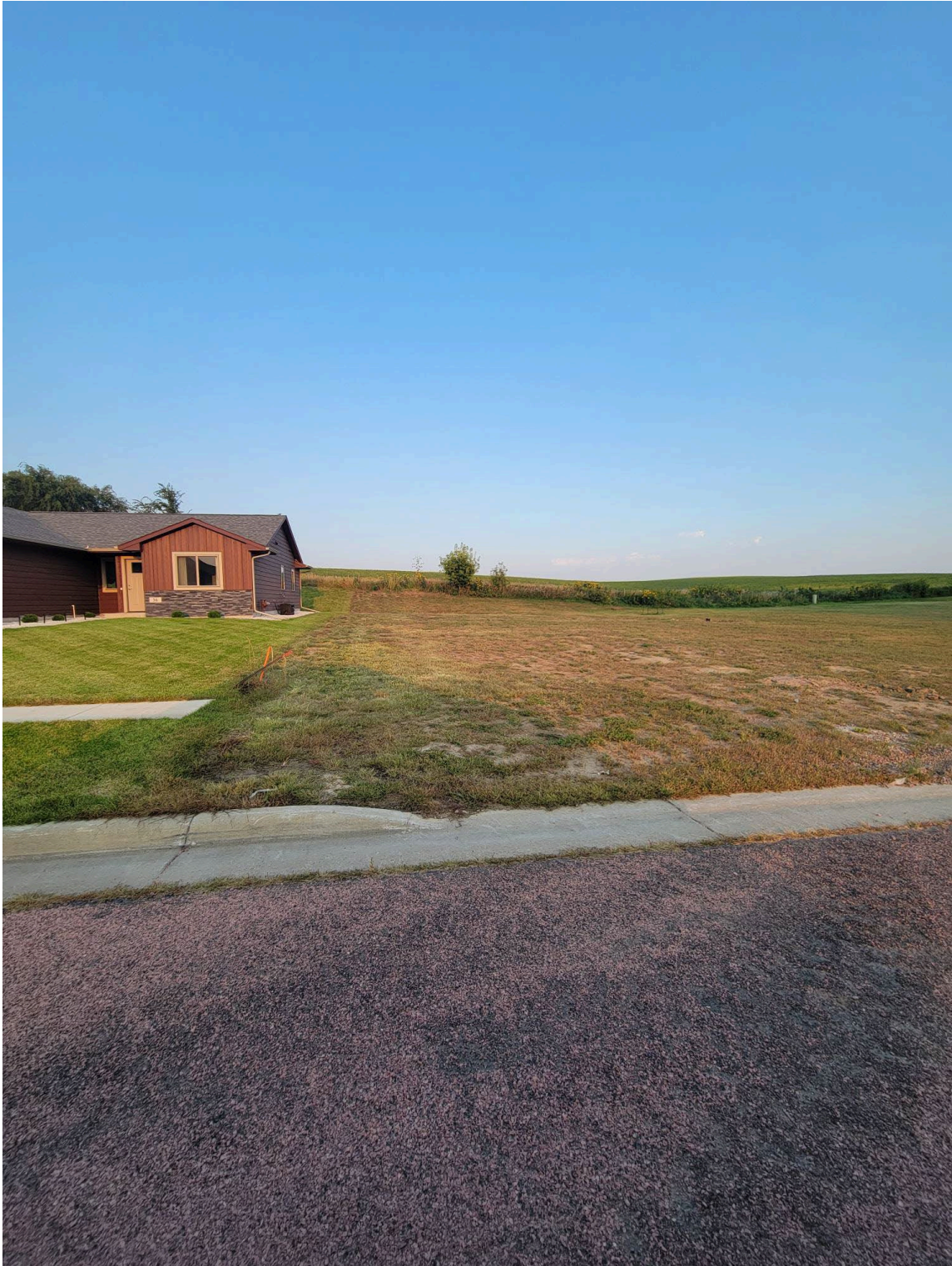
6 th Street facing west where the sidewalk ends
